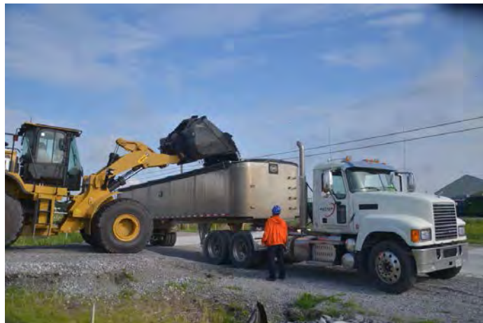
Figure 3.1 Transfer of the PGDP coal inventory to PACRO
