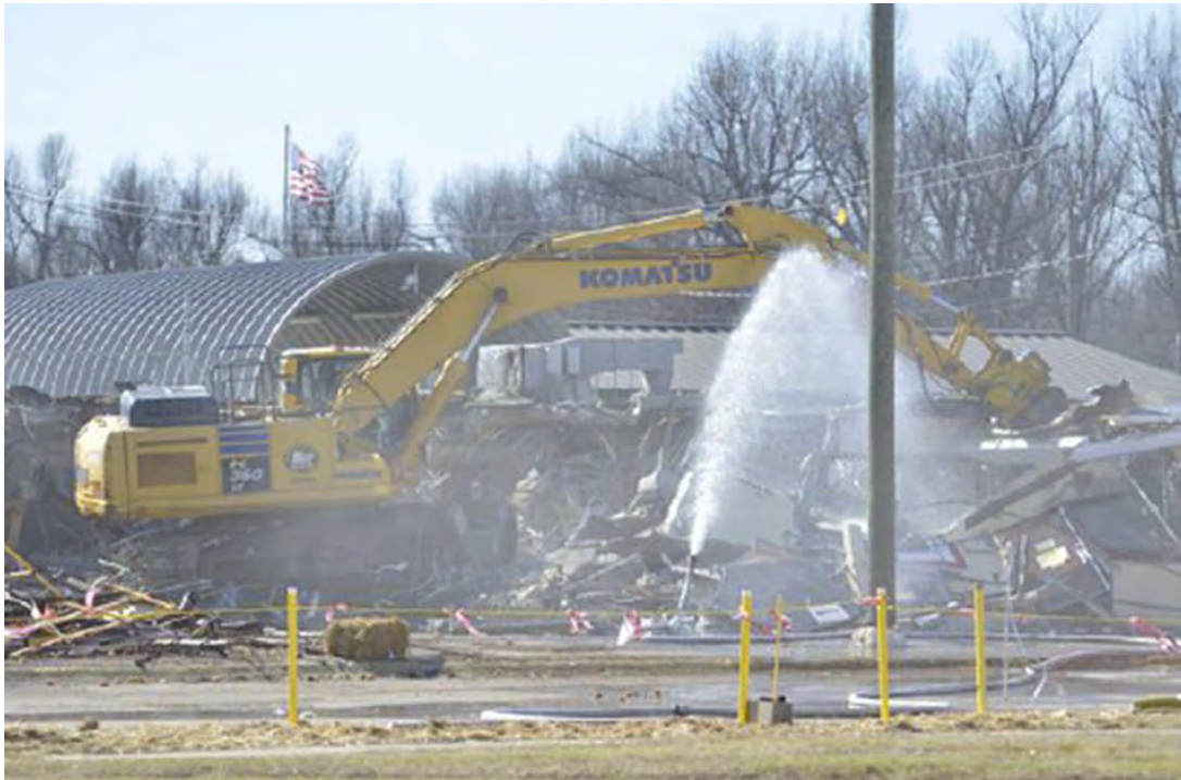
Figure 2.2 Demolition of C-212 Office Building
